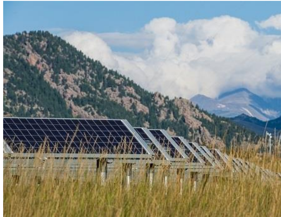
Sun Edison PV array at the NWTC. Photo by Dennis Schroeder, NREL 11249490
