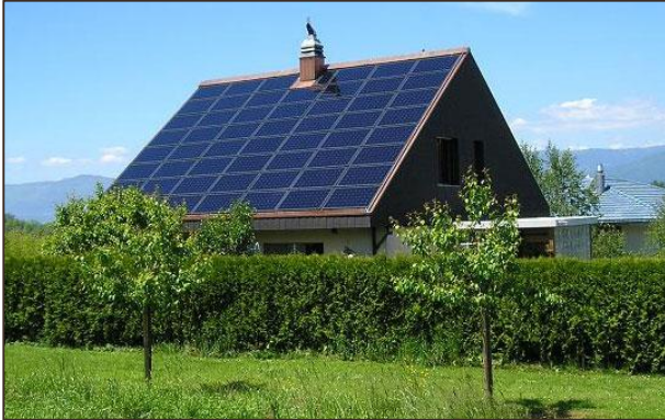
Solar Photovoltaic (PV)
